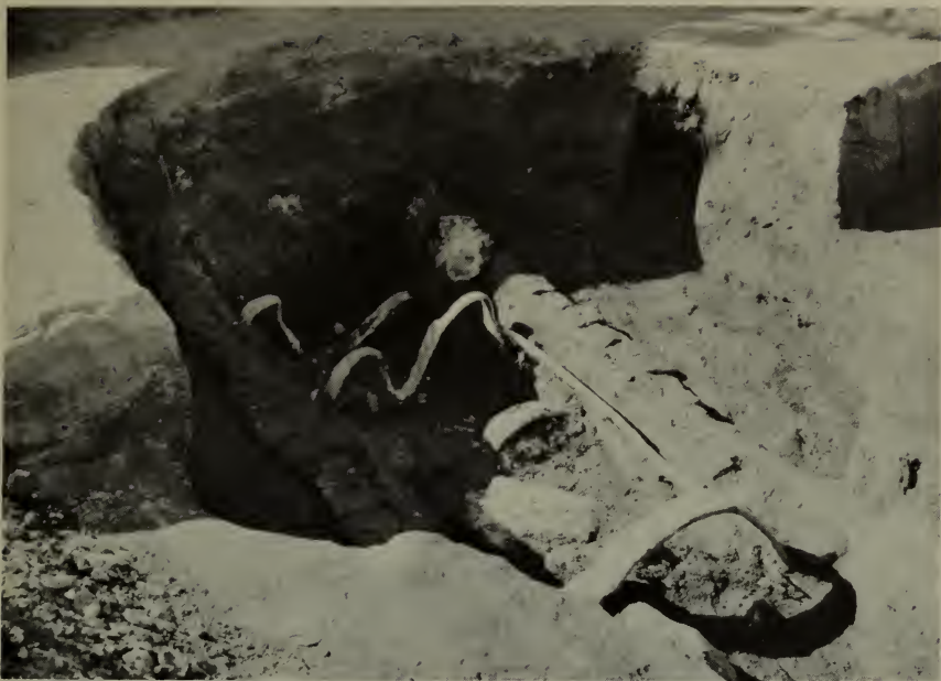
A 17TH-CENTURY LIME KILN EXCAVATED AT JAMESTOWN. IN IT OYSTER SHELLS FROM THE JAMES RIVER WERE BURNED FOR MAKING LIME. THE IRON HOOPS WHICH SUPPORTED THE ARCHED TOP OF THE KILN BUCKLED FROM THE INTENSE HEAT.
